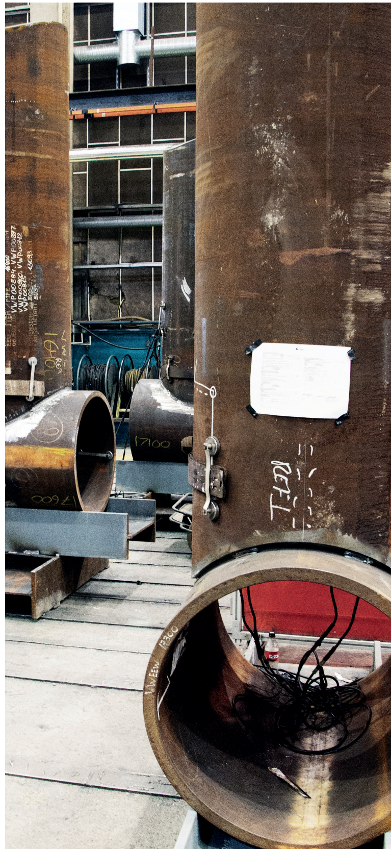
Pipe assembly hall at Aker Solutions in Verdal, Norway.
