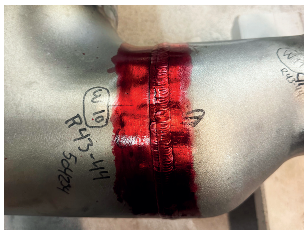
Penetrant testing on a weldseam
