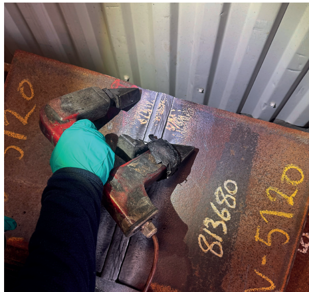
Magnetic particle testing on a weldseam
