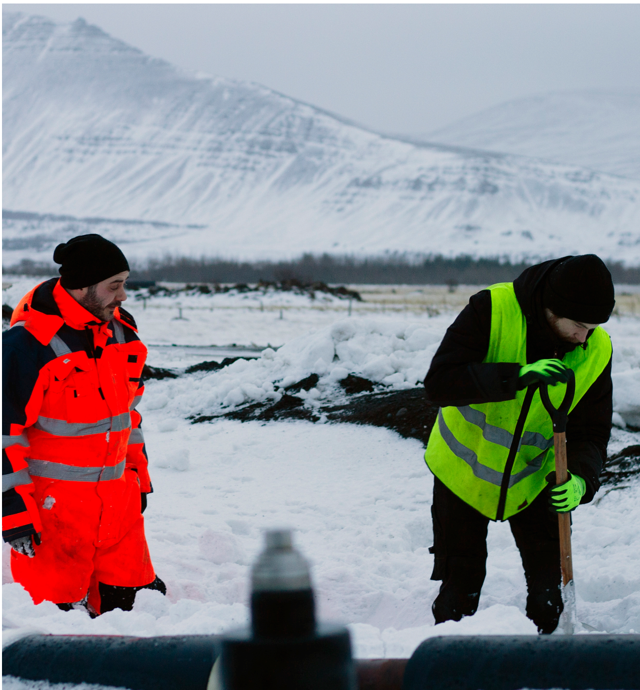
Andri and Magnús from HB Technology Services ehf., digging a central heating pipe free of snow for X-ray inspection.
