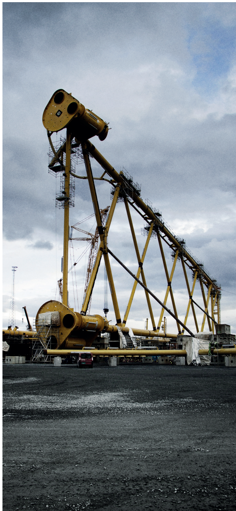
At the Verdal fabrication yard, jacket elements are assembled on the ground for offshore use.
