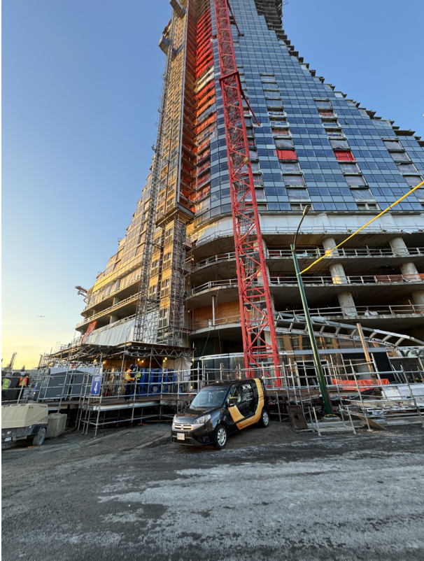
Oakridge shopping mall project for Ellisdon. X-raying for window installation pinning to avoid post-tension cables.
