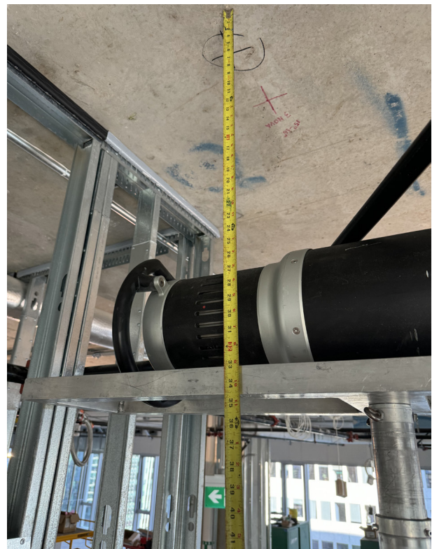
Comet X-ray EVO 300D setup at approximately 30" from underside of the slab.
