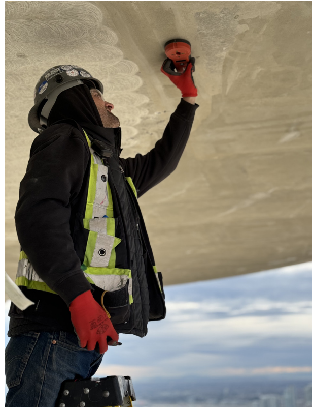
Nova technician using Hilti transpointer to locate core hole location on underside of slab.
