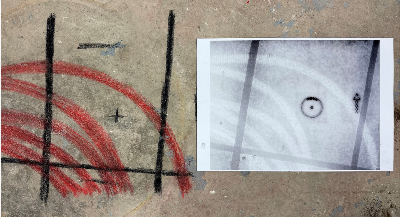
Detail slab analysis using both GPR scanning and digital X-ray.
